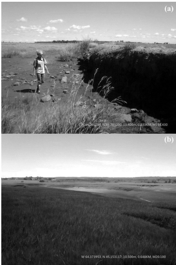
Figure 2: Geotagged photograph taken with the Trimble YUMA tablet during the ACAS shorezone characterization survey in 2011 at a) eroding dyke at Amherst Point, Cumberland Basin and b) extensive foreshore marsh protecting dyke at Kingsport, Cornwallis Estuary, Minas Basin.
